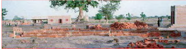
First buildings to be constructed include dormitories, dining facility and kitchen.
