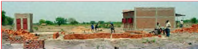
Preparing to lay foundation for guest house.
